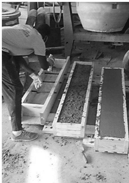
Fig. 6. Real data – case 1: Construction of the concrete box with three 19-mm reinforcing bars at depths ranging from 2.5 to 7.5 cm.
